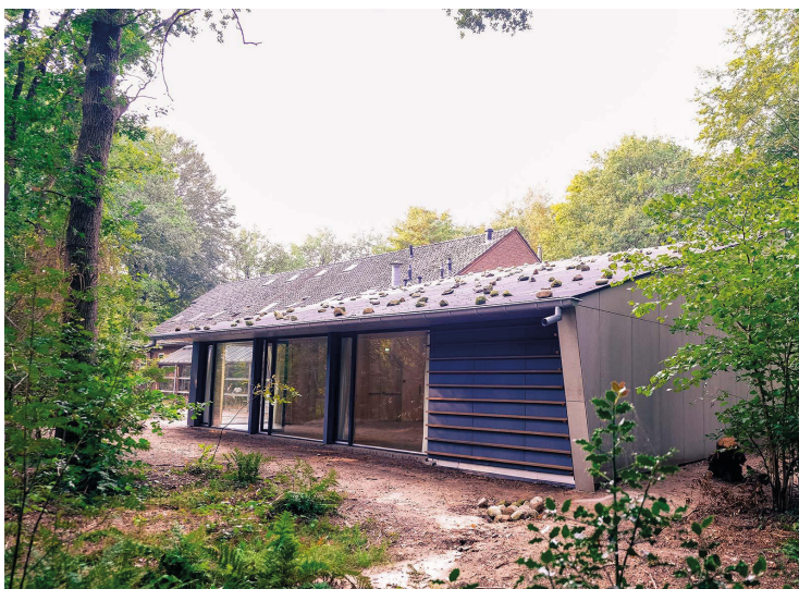
The 'Buitenzaal' with building 2 in the background
